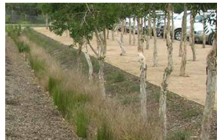
Water sensitive design techniques such as planted swales to treat stormwater run-off from car parks to be utilised
